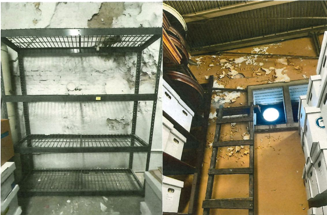
An example of falling plaster in the archives dept.'s mezzanine area (right wall) and paint peeling caused by moisture in the City Clerk's Records Room of the City Archives.
