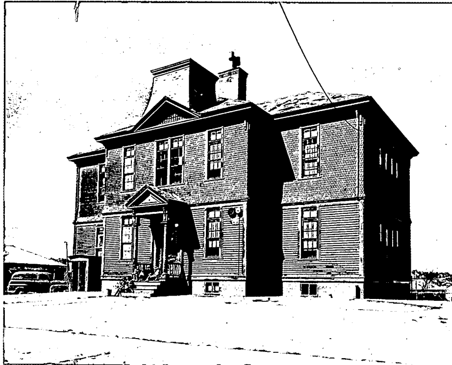
Nineteenth century schools were of two basic types of construction, all frame and frame with brick exterior walls. Still in use is Merino , one of three surviving all frame school houses.
