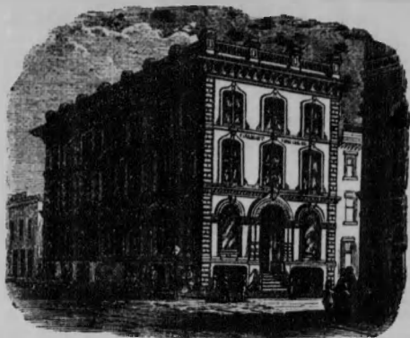
(Firemen's Fund Ins. Co.'s Building, S. W. cor. California and Sansom Streets, San Francisco.)
