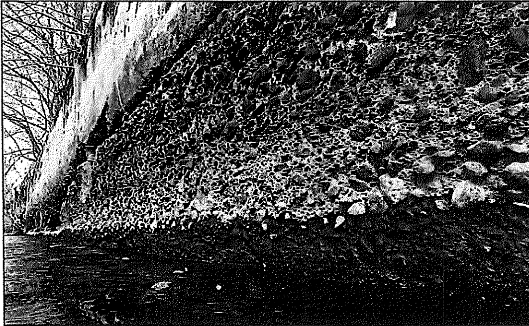
Photo 15: Typical scoured wall from waterline
