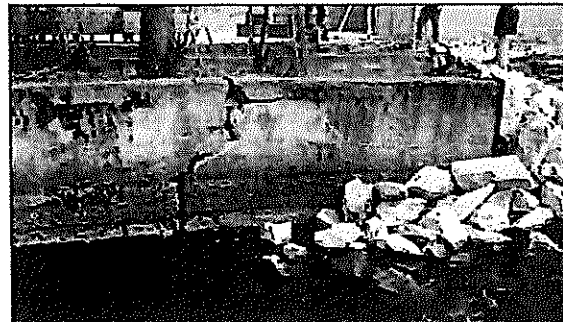
Large Crack at upstream end of concrete wall near Sta 2+00 and end of emergency repair.
