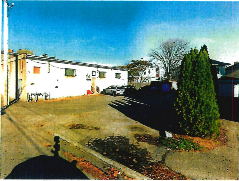
View of the site from Braman Street
