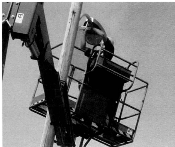
A PHA Electrical staff-person replacing site lights at Hartford Park
