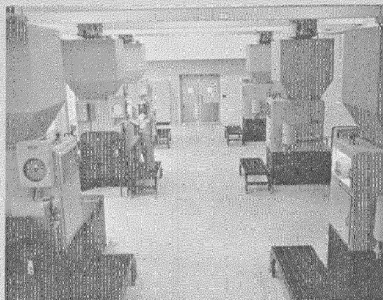
Introduction of chemicals into the treatment process is automatically controlled by modern chemical feeding machinery.
