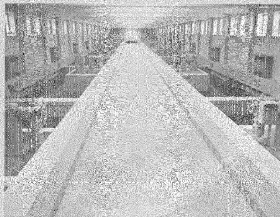
Filter gallery with electrically operated valves remotely controlled from Central Control Board.
