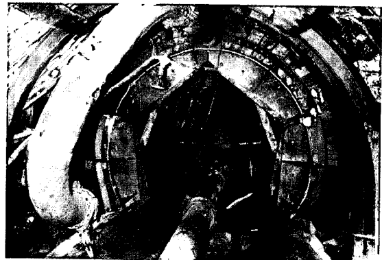
Forms in place ready to receive concrete lining in tunnel.
