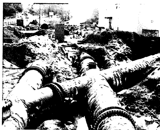
Manifold suction connection to the existing twin 60" steel pipe aqueducts showing the motor-operated valves that will be controlled from the centralized system at the Purification Works.
