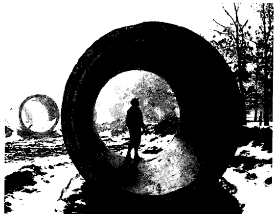
Project engineer inspecting 102-inch prestressed reinforced concrete pipe prior to installation.
