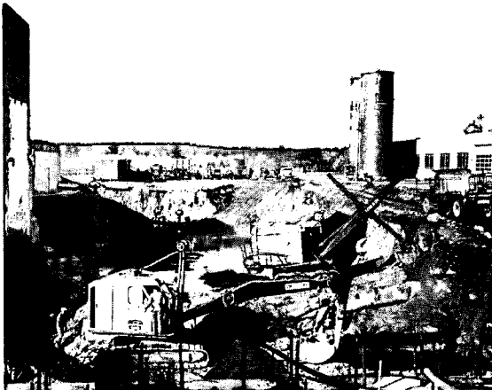
General excavation for filter plant extension that will increase capacity to 144 million gallons daily.
