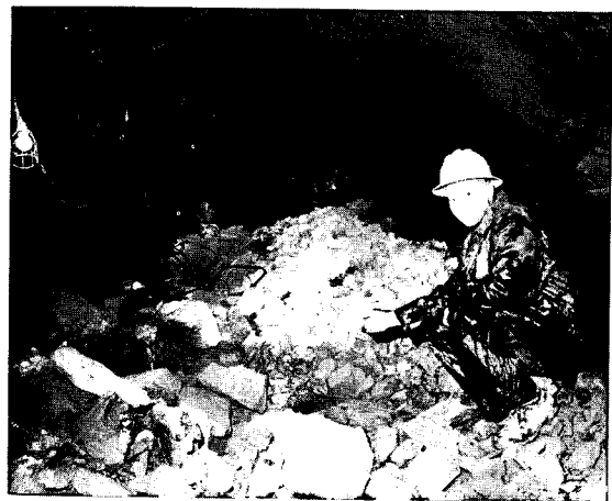
Rock spoil in tunnel immediately following blasting operations.
