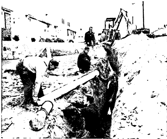
Distribution main being extended into residential development by private contractor engaged by the department through competitive bidding.
