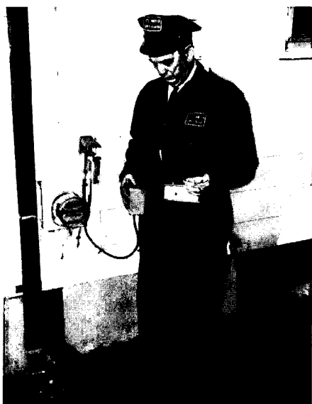
Meter reader inserts jack attached to visual recorder into outside receptacle in order to obtain remote reading on customer's meter.
