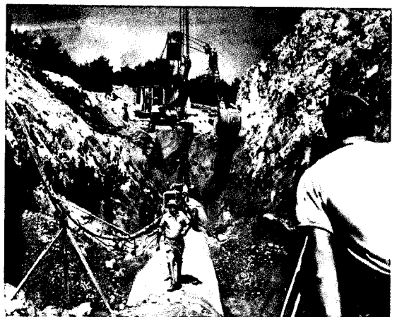
Department's field engineers checking alignment and proper bedding of pipe prior to backfilling operations.
