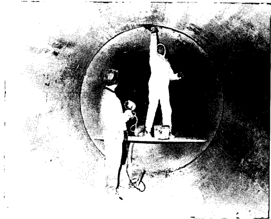
Pointing of interior joints of the installed pipe aqueduct section.
