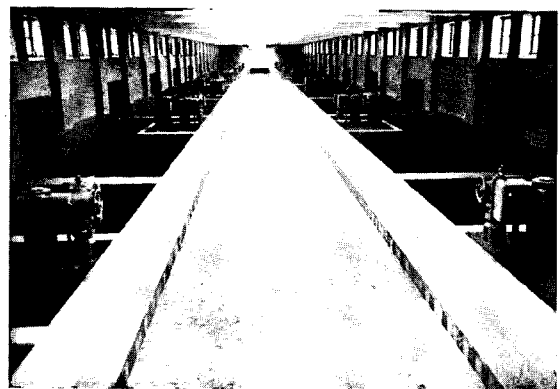
Filter gallery with electrically operated valves remotely controlled from Central Control Board.
