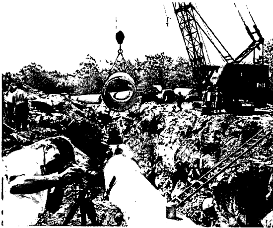
Work progressing on the installation of the 78" prestressed reinforced concrete steel cylinder pipe section of the Supplemental Tunnel and Aqueduct.
