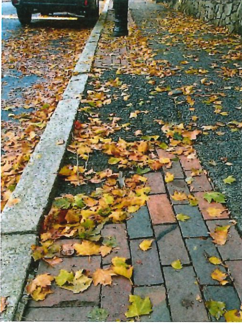
Brick border replaced by asphalt
