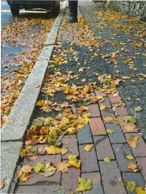
Brick border replaced by asphalt
