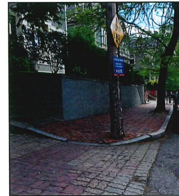
Sidewalk with steep grade.
