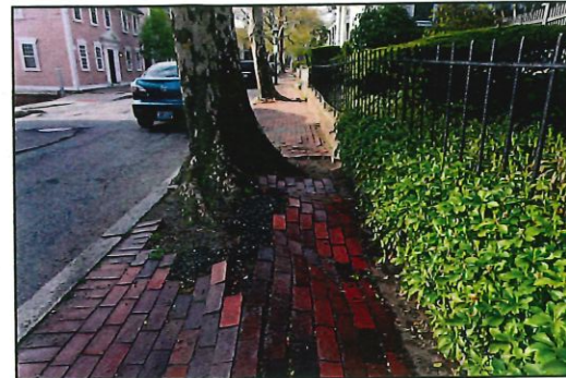
Impassable: Inadequate clearance and dislodged paving.
