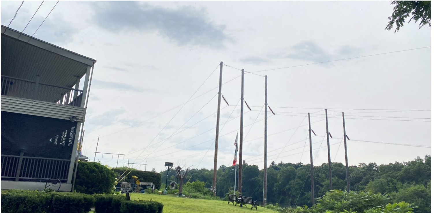
Photo #2: Existing conditions of 52 Ralston St. in Providence, RI.
