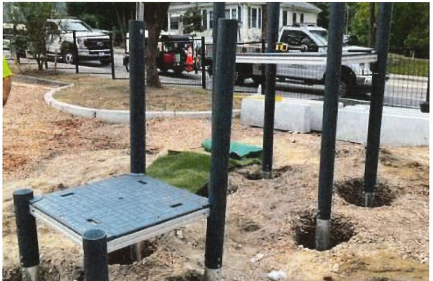
This image and below: Playground installation at Viscolosi Park.
