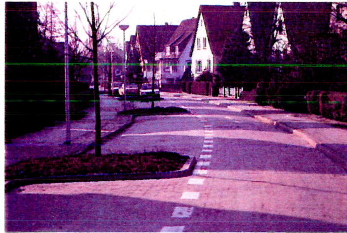
53. Tree planting brought out on one side but well into the carriageway, making yield movement inevitable next to every tree.
