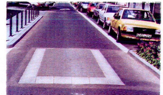
42. Speed cushions interrupt cars but allow larger vehicles to pass unhindered. They have to be either side of an at-grade crosswalk, Cologne, Germany. (Photo: Paul Murrain)
