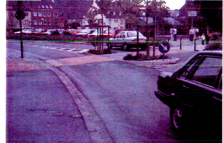
54. A central island narrowing a carriageway. In this case, it incorporates a crosswalk. Jülich, Germany. (Photo: Graham Paul Smith)
